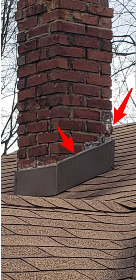
Counter flashing should be installed into mortar joints
