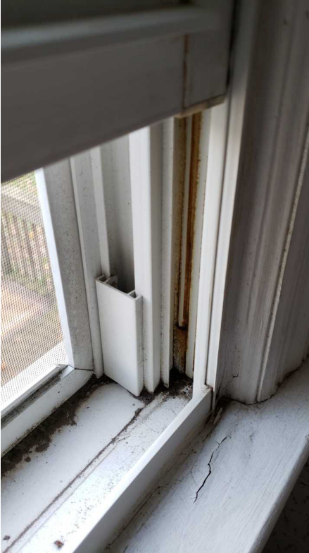
Window doesn't remain open. Broken latches
