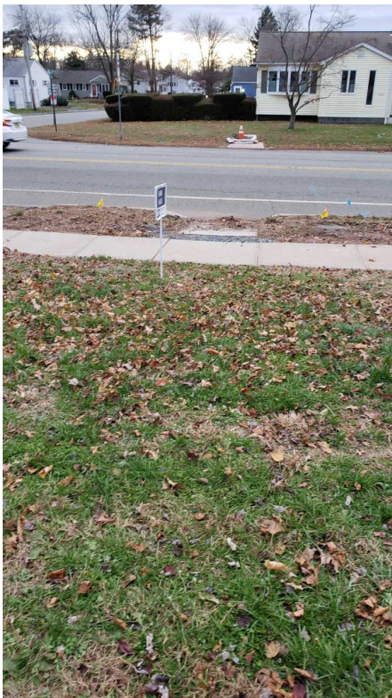
Gas line markout and asphalt patches located in front yard and sidewalk of the property
