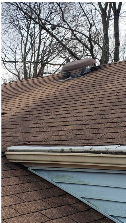
Gutter slopes towards roof
