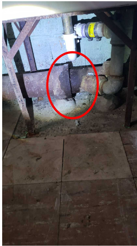
Corrosion on supply lines in kitchen
